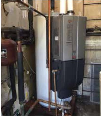
Internal testing showed that the Demand Duo™ system on average produces 338 gallons of hot water in the first hour, compared to a standard efficiency tank's 248 and a high-efficiency tank's 315. For the restaurant, this high-performing difference was the much needed solution for the business and its customers.
